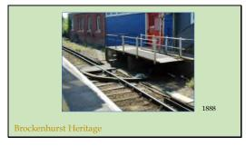
Another 1888 innovation was this – a traverser bridge. Other than the stairs there was no way onto the platforms which for parcels or porters with trolleys was a nuisance. So, this bridge was installed, which could be swung out over the tracks by the ticket office to at least provide access to platforms one and two.
